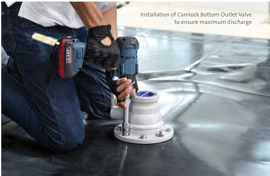
Installation of Camlock Bottom Outlet Valve to ensure maximum discharge
